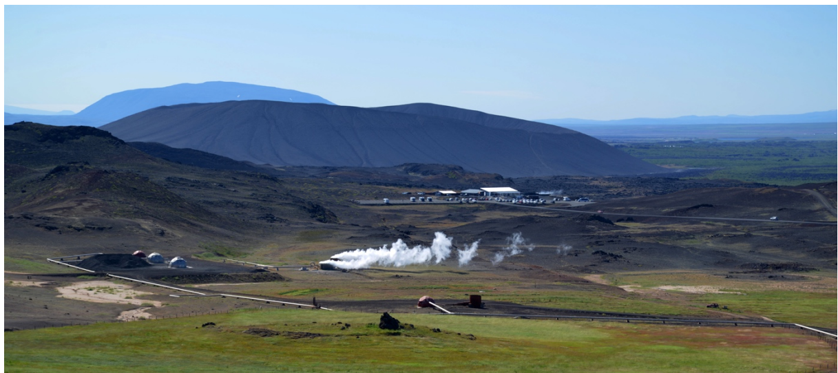
Geothermal power plant in Iceland
