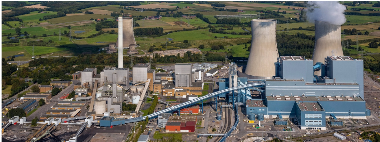
Coal fired power plant in Germany
